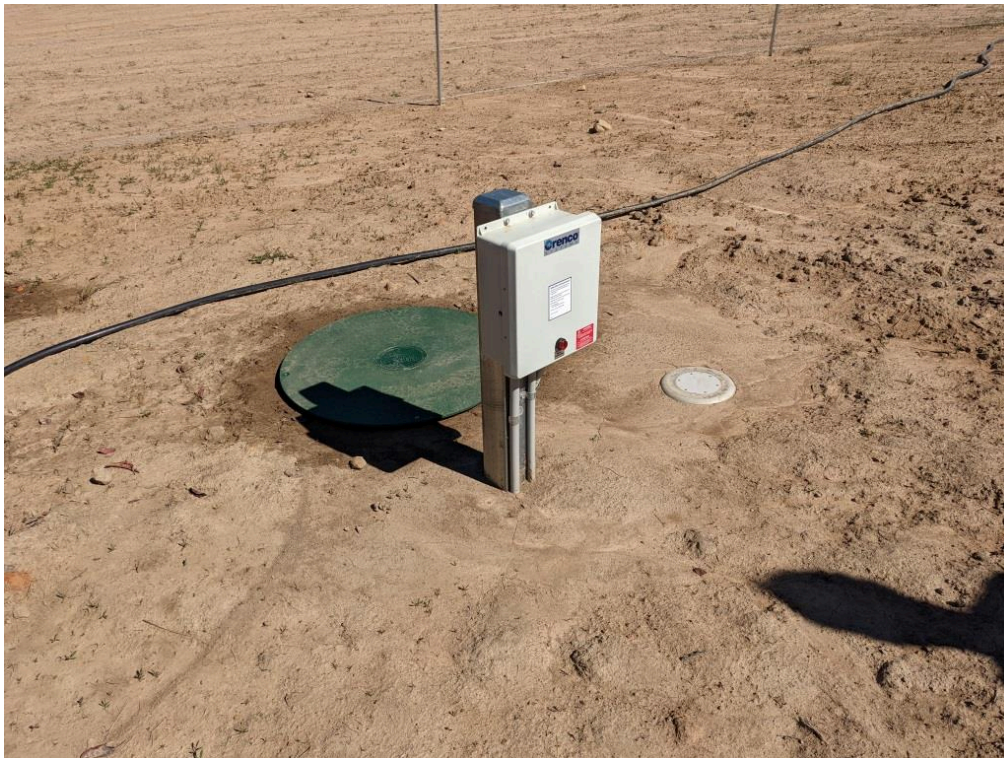
Figure A.3.1 On-property STEP tank installation.
