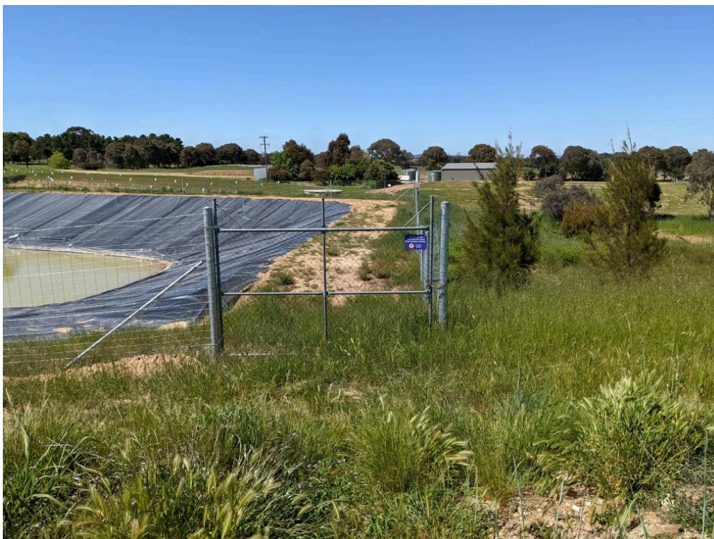
Figure A.3.6 Wet weather storage is enclosed within security fencing; recycled water signage at point of entry.
