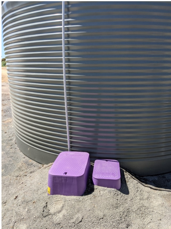
Figure A.5.3 Valve pits adjacent to the treated effluent tank coloured lilac/purple; and Flushing pit in the irrigation area coloured purple and clearly labelled.
