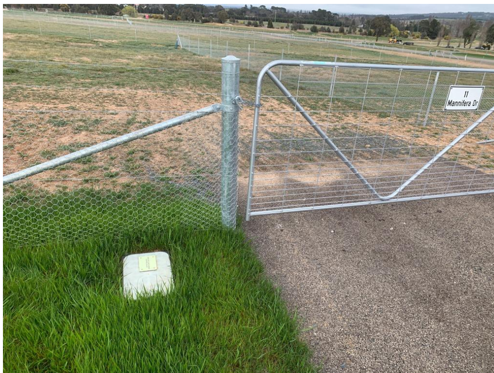
Figure A.9.6 Re-established (grassed) surface around property service connection box within road reserve.
