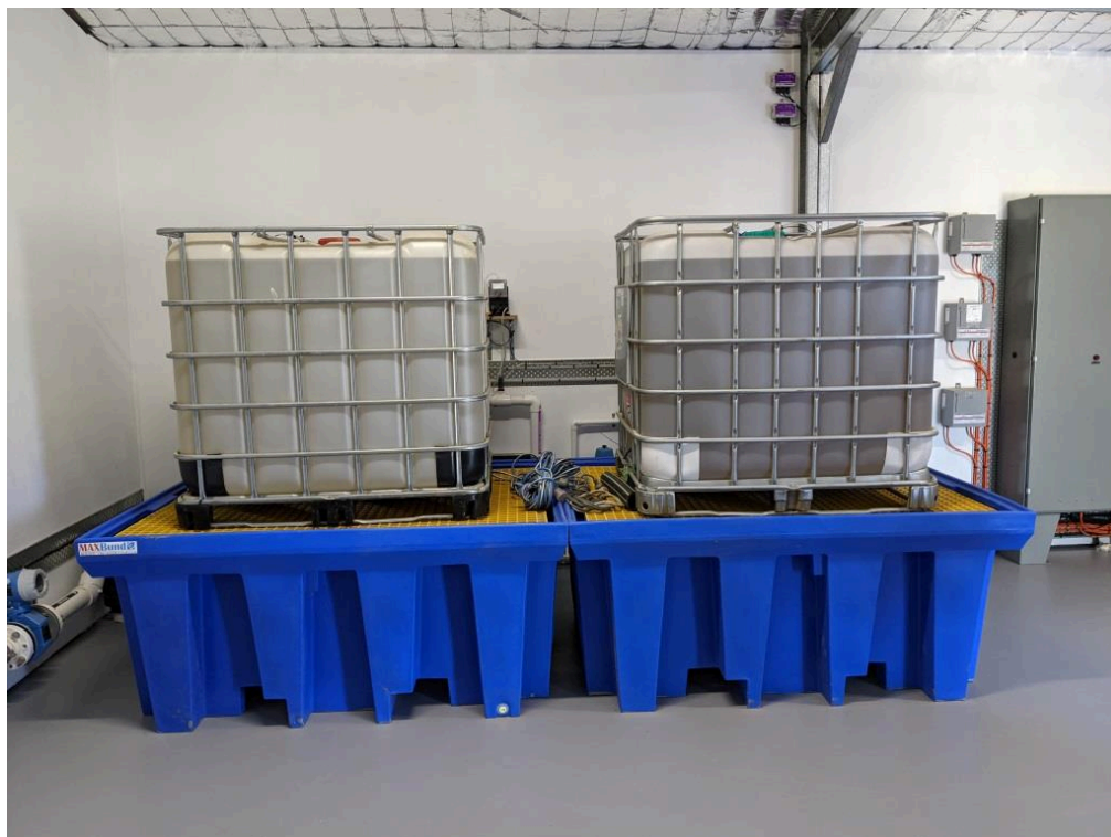
Figure A.5.4 Chemicals are stored over over bunded areas (grated top tanks).
