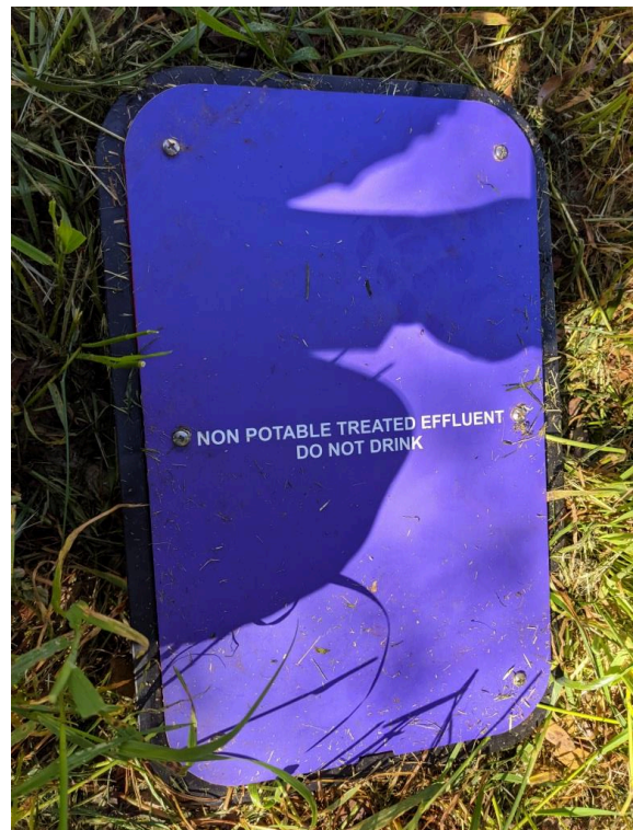
Figure A.5.3 Valve pits adjacent to the treated effluent tank coloured lilac/purple; and Flushing pit in the irrigation area coloured purple and clearly labelled.
