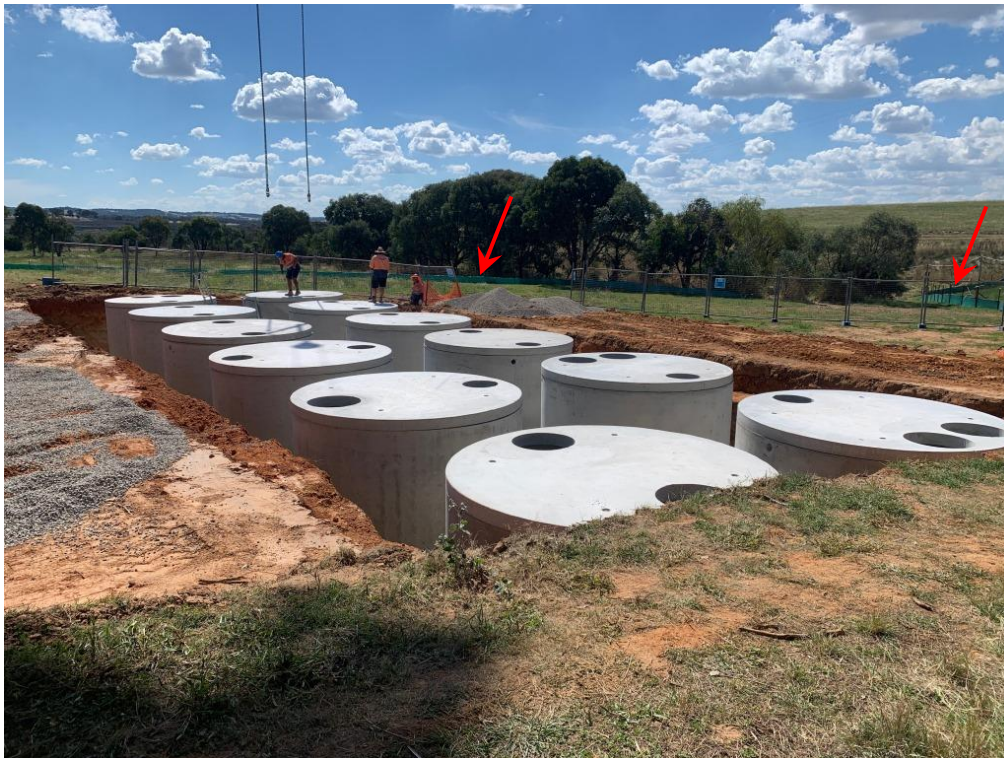
Figure A.9.1 Treatment plant construction showing silt fencing (arrowed) in background.
